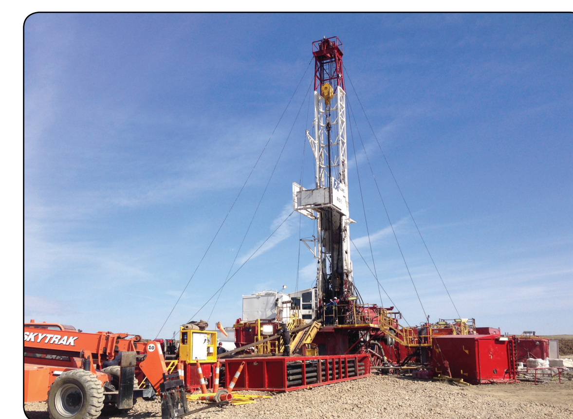
Drilling first CO 2 production well
